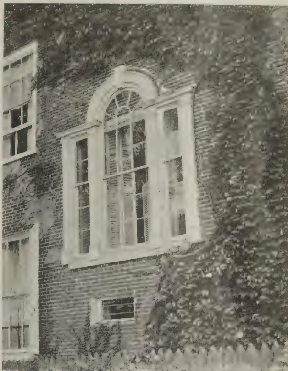
FIG. 2. REED HOUSE, NEWCASTLE, DEL. BUILT 1801
